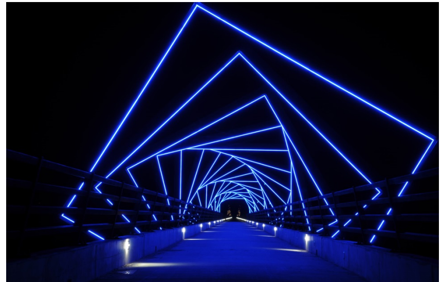
High Trestle Trail, Madrid/Woodward
